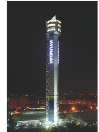
Hyundai Asan Tower The World's Highest Elevator Test Tower (Hyundai Asan Tower) stands in Icheon, Korea
