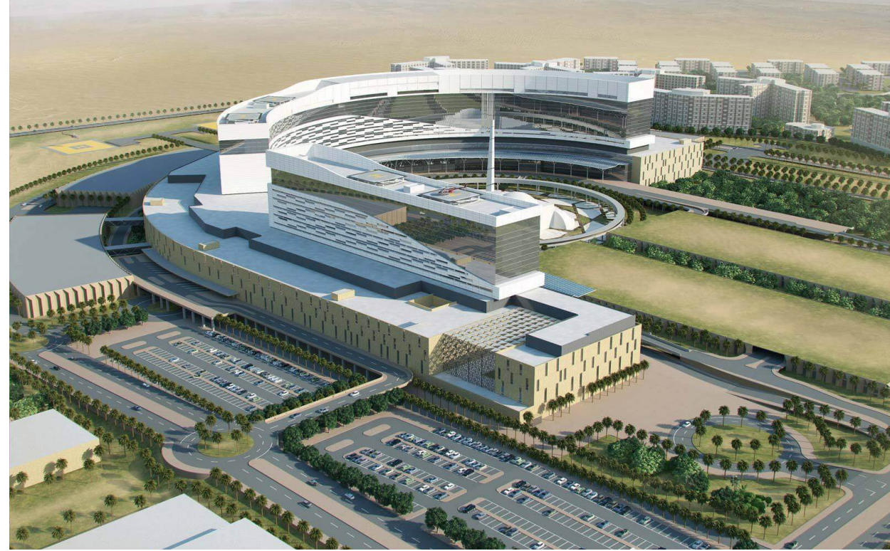
← 사우디아라비아 Security Forces Medical City MAX. 150m/min 284 elevators 24 escalators
