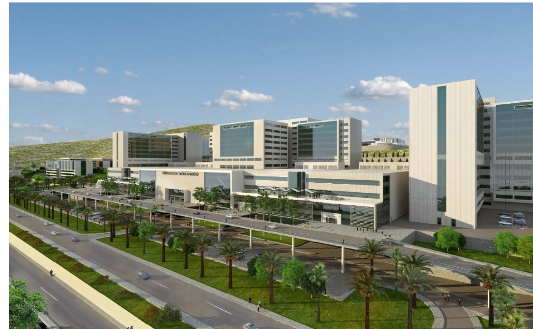
↑ 터키 Izmir Bayrakli Integrated Health Campus MAX. 105m/min 110 elevators 20 escalators
