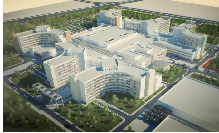
↑ 터키 YDA Konya Hospital MAX. 105m/min 72 elevators 42 escalators
