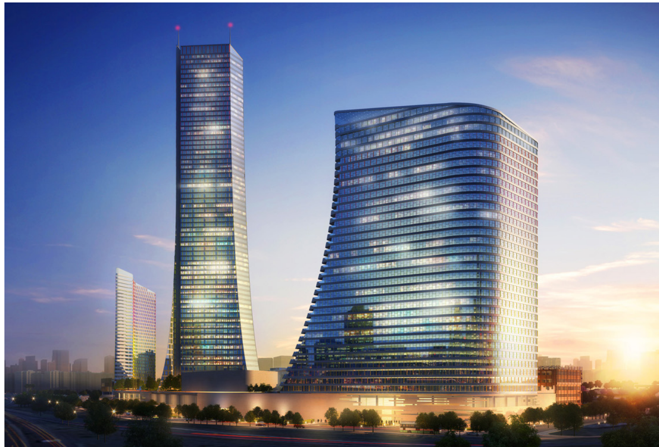
↓ 터키 Metropol MAX. 360m/min 99 elevators 29 escalators
