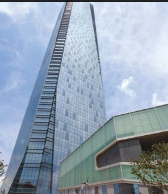
Busan International Finance Center (BIFC) | Busan, Korea [High-speed elevators] 600m/min., 2 units | 540m/min., 3 units | 480m/min., 8 units | 46 units in total
