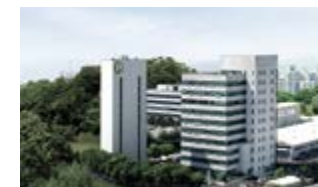
Icheon Head Office (Gyeonggi-do) | [Factories 1, 2 and 3] Advanced production facilities (46,484m 2 ) | Manufactures elevators, material handling systems, parking systems and platform screen doors (PSD)
