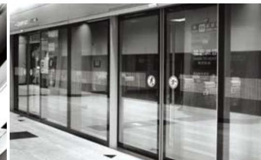
Platform Screen Door
