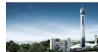
Hyundai Asan Tower | The tallest elevator test tower in the world
