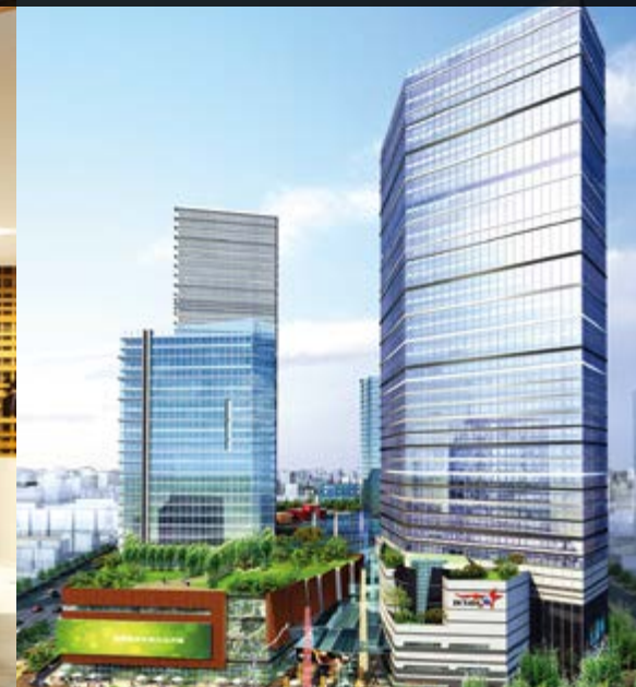
Lerthai Center | Shijiazhuang, China 360m/min., 4 units | 10 units in total
