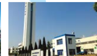
China Factory (Shanghai, China) | Scale: 28,716m 2 | Manufactures elevators and escalators | Elevator test tower (height: 72m)
