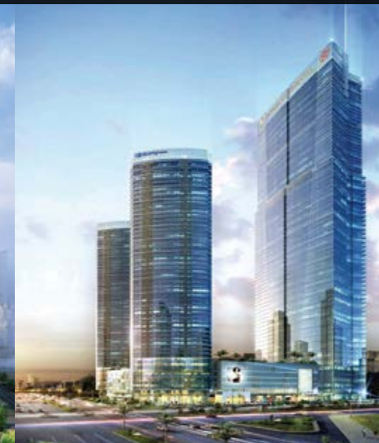
Hanoi Landmark Tower | Hanoi, Vietnam 240m/min., 2 units | 29 units in total
