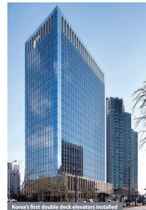
Korea's first double deck elevators installed
