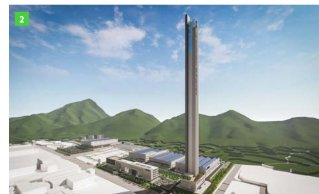
1. Manufacturing of elevator doors 2. Aerial view of a new Chungju factory
